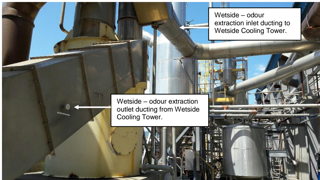
Wetside Process Vapours to Wetside Cooling Tower
